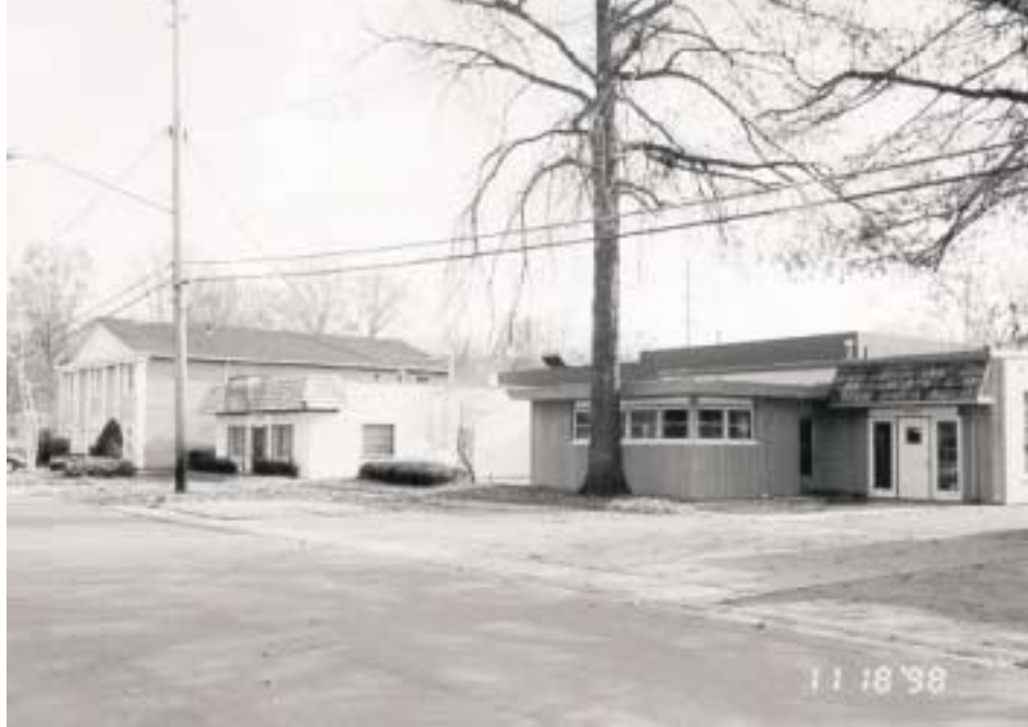
Vacancies and the appearance of the buildings on the south side of Knickerbocker detract from the character of the area. The City's senior resident apartment building is located across the street.
