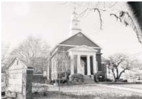
Bay Village City Hall, originally constructed in 1914, also houses the City's police department. Due to a lack of space, the City is studying whether to expand City Hall or build a new police station.
